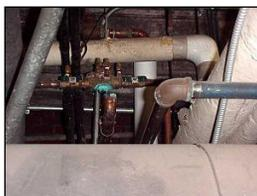
**Back flow preventor** showing scale buildup on drain opening may indicate the back flow preventer needs to be tested for proper operation.
