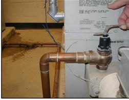
**Manual test of relief valve.** The manual test lever on the relief valve should be lifted on a regular basis to determine the valve is functioning properly. The pressure in the boiler should be at least 75% of the set pressure of the relief valve.
