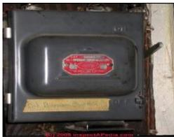
**A manually operated remote shutdown switch** or circuit breaker shall be located just outside the boiler room door and marked for easy identification.
