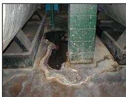
**Water and scale buildup** on floor indicates the relief valve has been leaking past seat for some time. This valve should be replaced as soon as possible as it could scale up and become inoperative.
