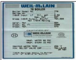
All boilers that are required to have **operating certificates** shall have a manufacturer's nameplate attached. The nameplate shall have the appropriate ASME Code symbol, the allowable working pressure, date of manufacture, and the minimum relief valve capacity.
