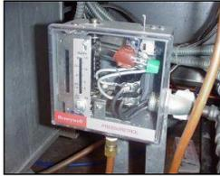
**Pressure control showing mercury switch and manual reset on top.** (Warning: Care should be taken with mercury switch as the mercury is highly toxic and any spills must be reported to the proper authority. Cleanup of a spill can be very costly.)
